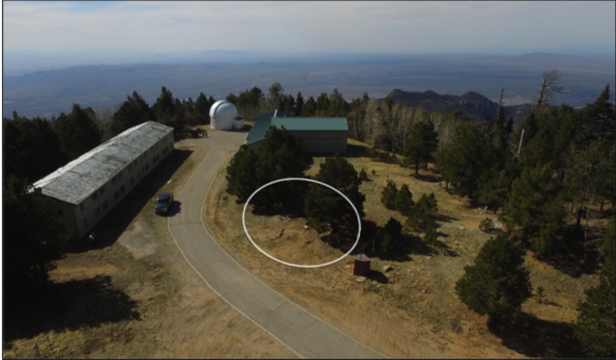
Figure 8. The prime location for the first ATO on Mt. Lemmon, on the ridge just west of the old Air Force Station radar tower. The large building on the left (Army barracks) is planned to be removed from the site.
